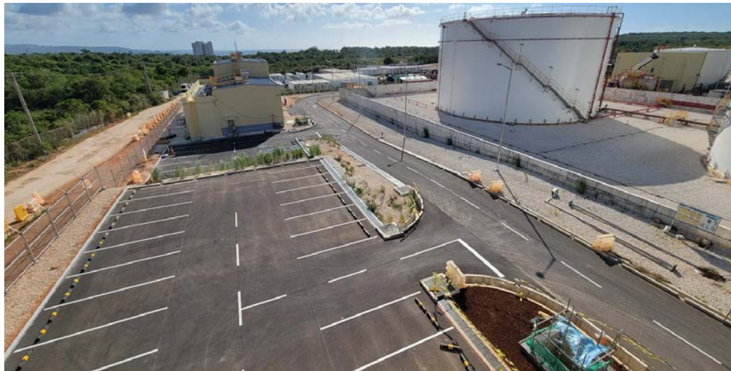
Parking lot near Admin building has been completed
