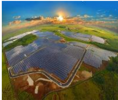
Dandan Solar 25 MW Ph I
