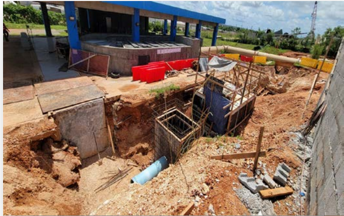
Motorized Valve Pit Forms with Piping
