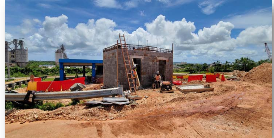
Rebar installation is ongoing in Communications Room
