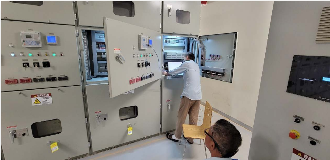
Testing inside BESS Control Room
