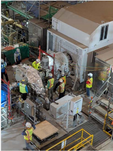
Alignment between HP turbine and generator
