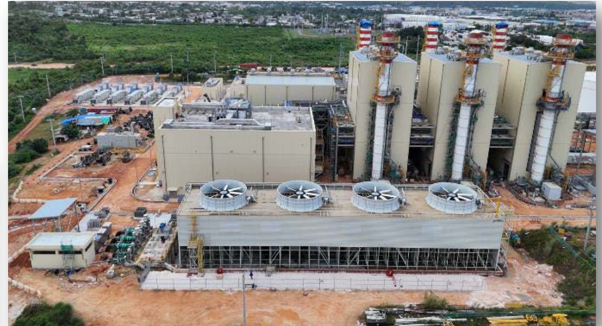
Cooling Tower & Basin – Commissioning work is ongoing.
