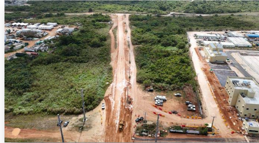
Access road ground compaction and asphaltting in progress
