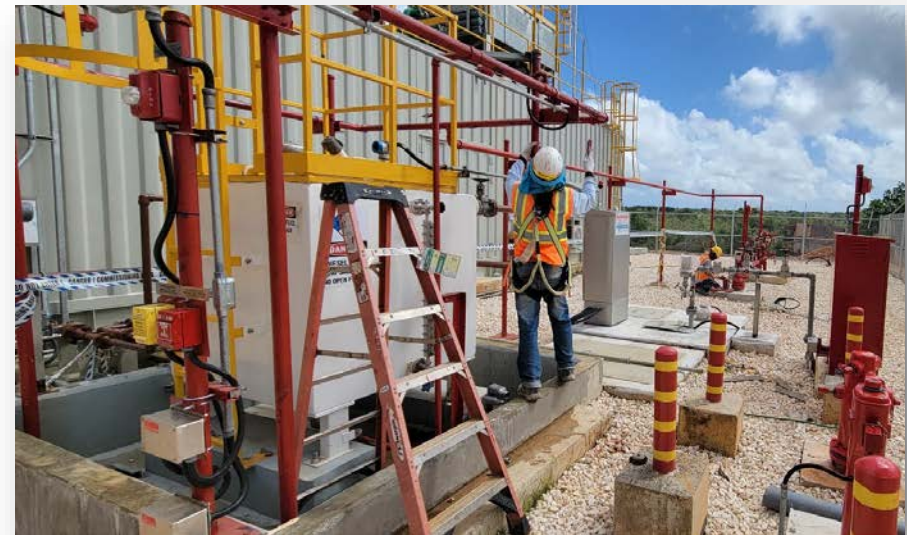
Painting ongoing of fire suppression piping
