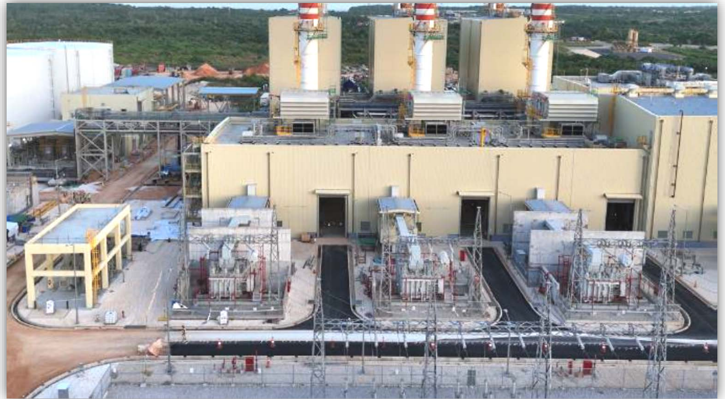
GTG Building – Commissioning work is ongoing.
