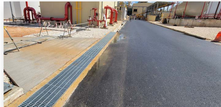
Installation of grating over storm water ditches is ongoing
